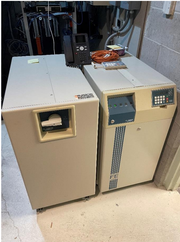
← Uninterrupted Power Supply – UPS
